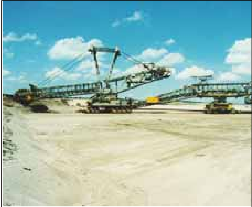
Laubag open-cast mine at Nochten, bucket wheel excavator SRs 6300 + loading unit VR 156.12 equipped with 50 ELHY units
